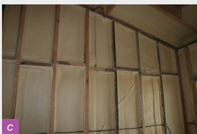
Figure 2: Applications of polyurethane spray foam (SPF) a) installed under a timber floor (photo courtesy of Pacific Urethanes Pty Ltd), b) being installed to the inner masonry leaf prior to installing the external brick veneer (photo courtesy of Huntsman Polyurethanes Australia), c) being installed in Melbourne as cavity insulation prior to the plasterboard (photo courtesy of Huntsman Polyurethanes Australia).
