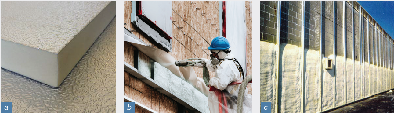
Figure 1: a) PIR board insulation with foil facers (photo courtesy of Pirmax Pty Ltd), b) Installation of polyurethane spray foam to a wall (photo courtesy of Huntsman International LLC), c) Installation of ccSPF to a concrete block wall (photo courtesy of Huntsman Polyurethanes).
